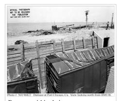
Boxcars within their revetments near the pier were crushed by the pressure of the blast.
