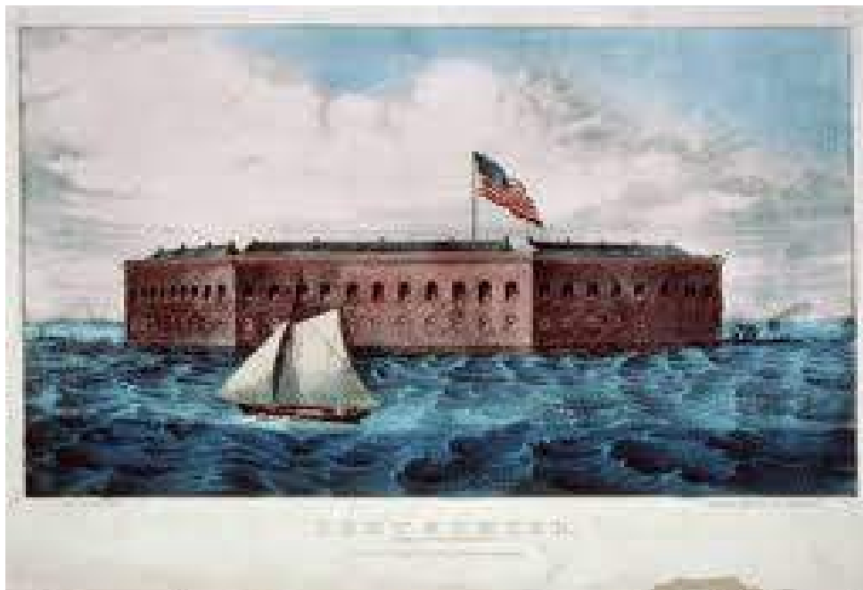
Fort Sumter, South Carolina
